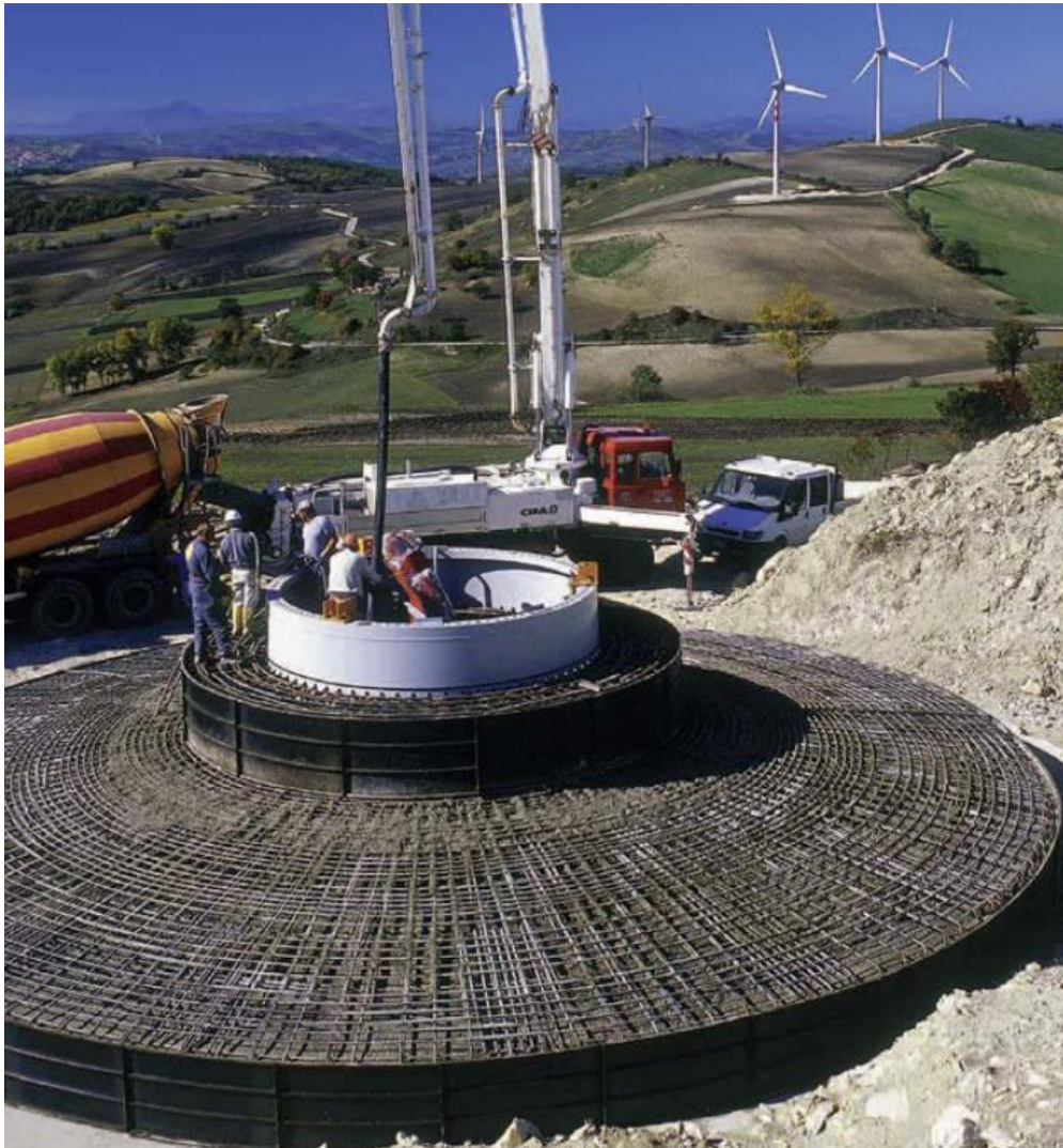
Plate 3.2: Wind turbine foundation 6
