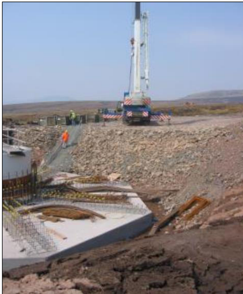
Plate 3.1: Turbine foundation under construction with adjoining crane pad 5
