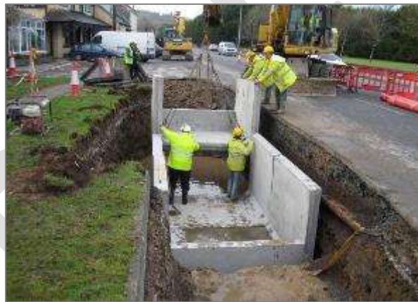
Figure 8 – Example of Joint Bay under construction (pre-cast)
