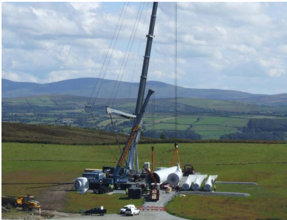
Plate 3.3: Wind Turbine Erection 2
