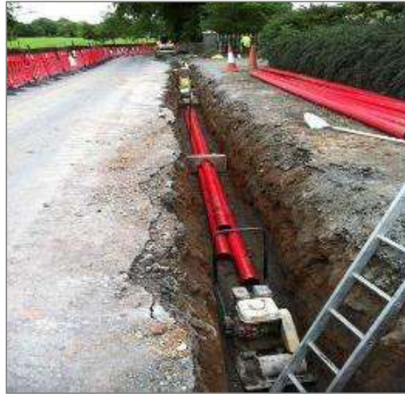
Figure 2 – Example of 110kV Underground Duct Installation
