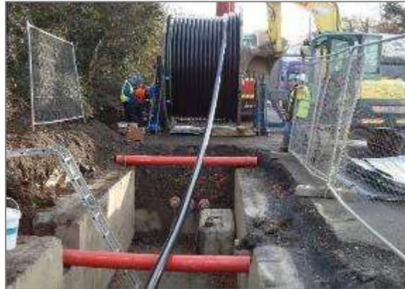
Figure 9 - HV cable pulling procedure (Drum set-up example)
