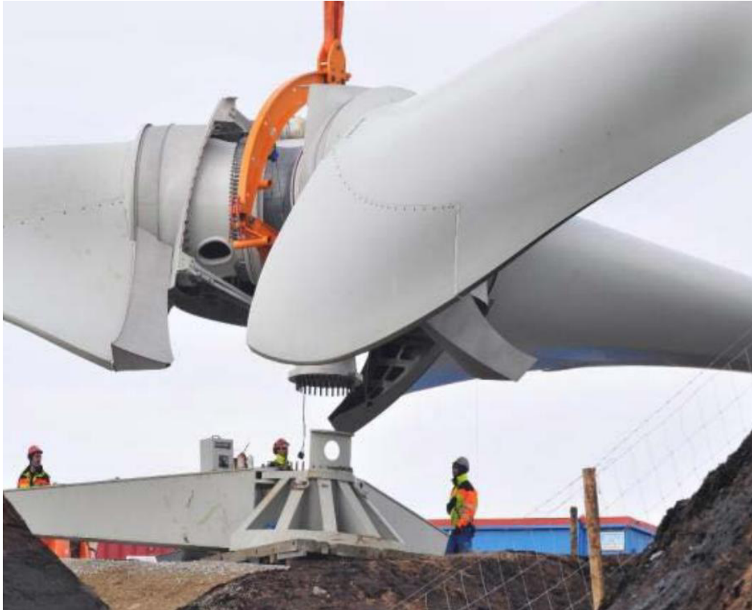
Plate 3.4: Assembly of wind turbine blades 2
